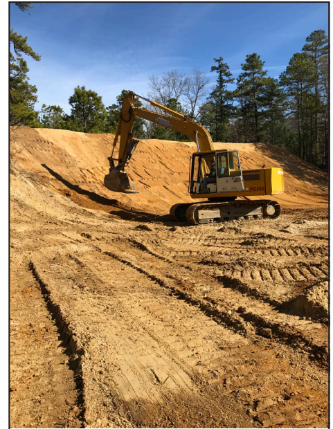
Construction work on the pistol berm.
