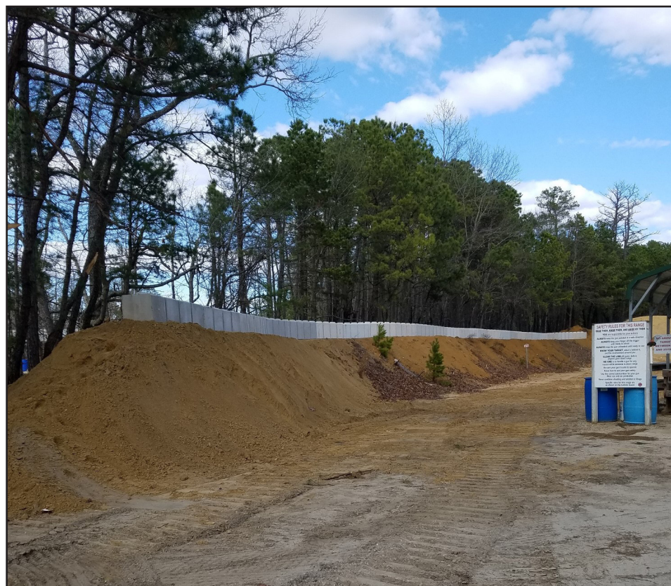
Extended and improved side berm on the plinking range.
