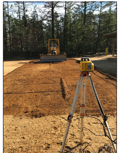
Grading for drainage on the pistol range.
