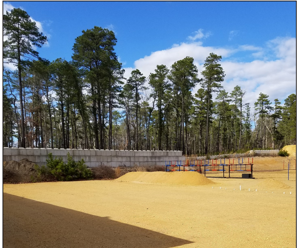
Greater height added to the side berm on the pistol range.
