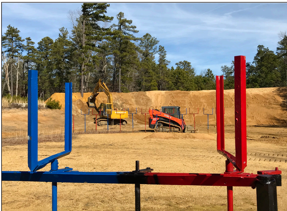
Rebuilding the pistol range berm.
